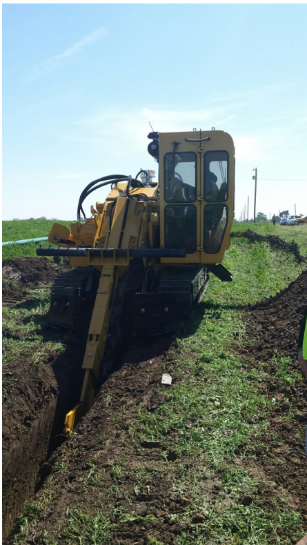
The trench being cut for the new 8" steel pipeline.
