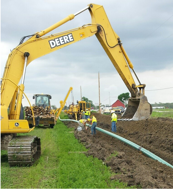
New 8" steel is lowered into the trench by Miller Pipeline.
